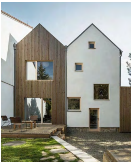
Double gable house, Pro story, Tjeckien
